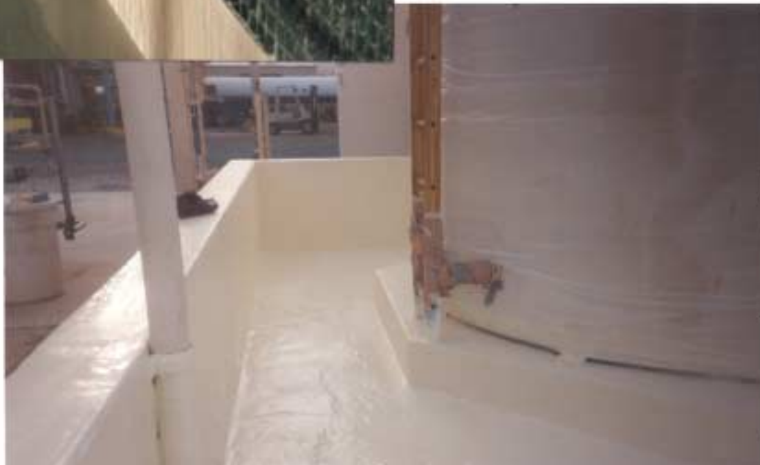
View of EF-1990 applied as secondary containment lining system for hydrofluoric acid. EF-1990 was applied as an ECOSYSTEM ® expanded film for sealing the rough concrete floor followed with a solid topcoat for added strength.
