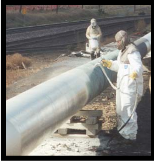
Field application of EF-RBU over FBE Blasted to SSPC-SP7 "Brush-Off " Blast
