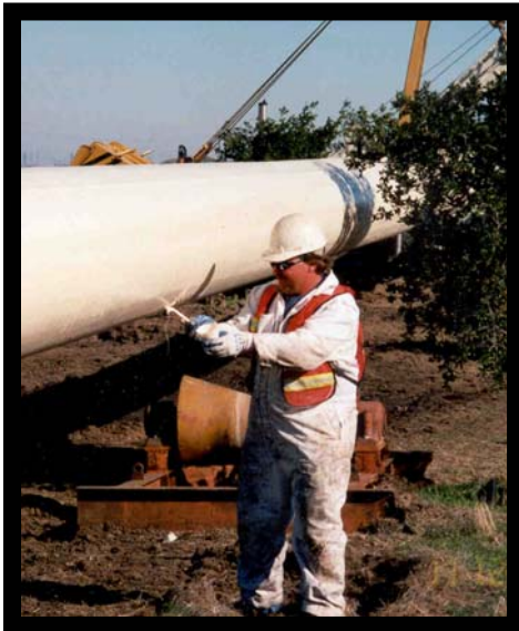
View of field repair to EF-RBU
