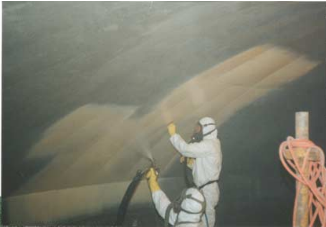
View of direct-to-concrete application of EF-1990 to interior of a water storage vault utilizing plural component spray equipment.
