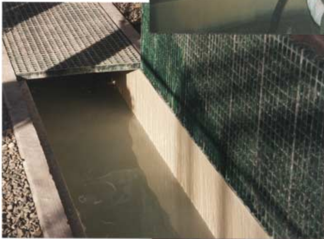
View of direct-to-concrete application of EF-1990 to interior of a water storage vault utilizing plural component spray equipment.
